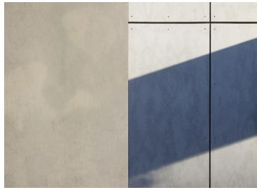
2. PREFINISHED CONCRETE CLADDING WITH EXPRESSED JOINTS
